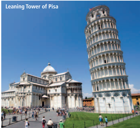
Leaning Tower of Pisa
